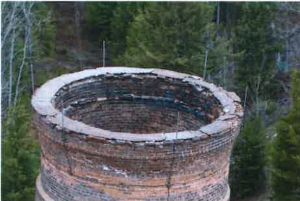
Figures 7 (left) and 8 (right) – Top of the chimney. Note loose bricks and mortar in imminent danger of falling.
