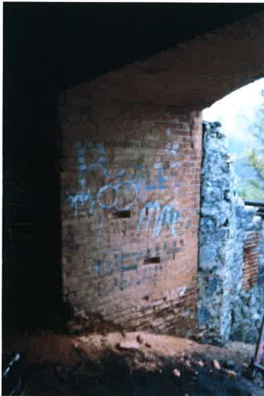
Figure 3 (left) – Interior of the chimney
