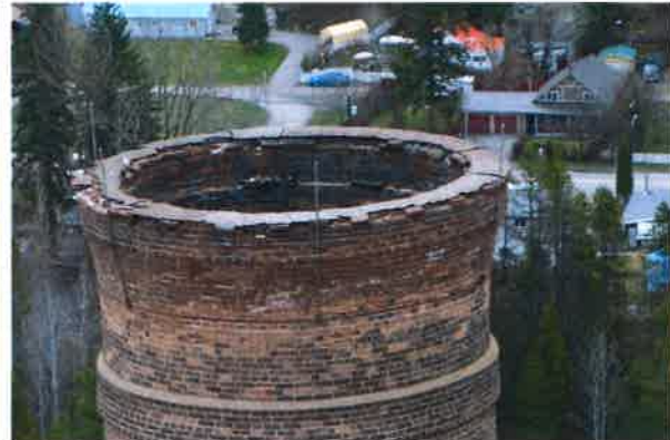
Figures 7 (left) and 8 (right) – Top of the chimney. Note loose bricks and mortar in imminent danger of falling.
