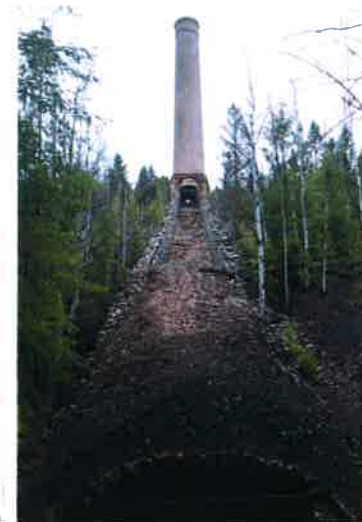
Figure 2 – General view of the smelter's flume and chimney
