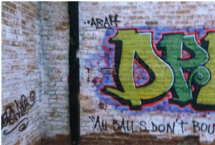
Figure 15 – Location and brick #2 (Corner building)
