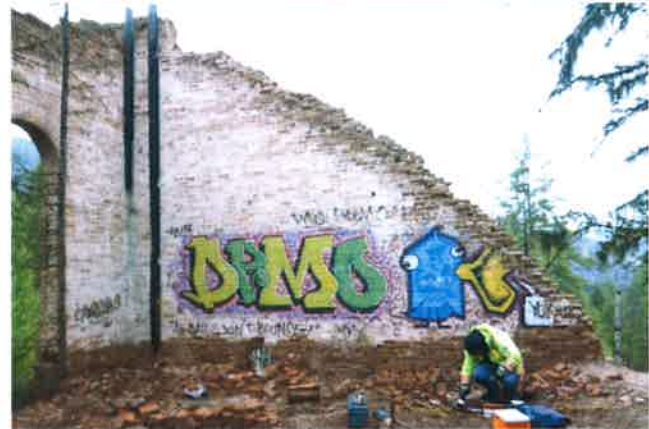
Figure 6 (right) – South view of the Corner Building wall.
