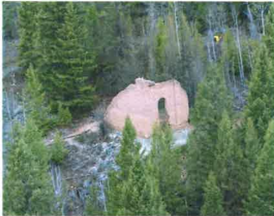
Figure 5 (left) – Aerial view of corner building.
